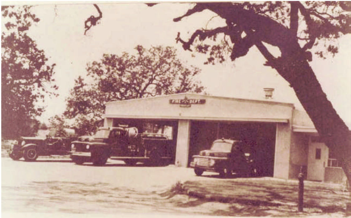
New Erbes Road Station 31 - 1949 to 1977.
