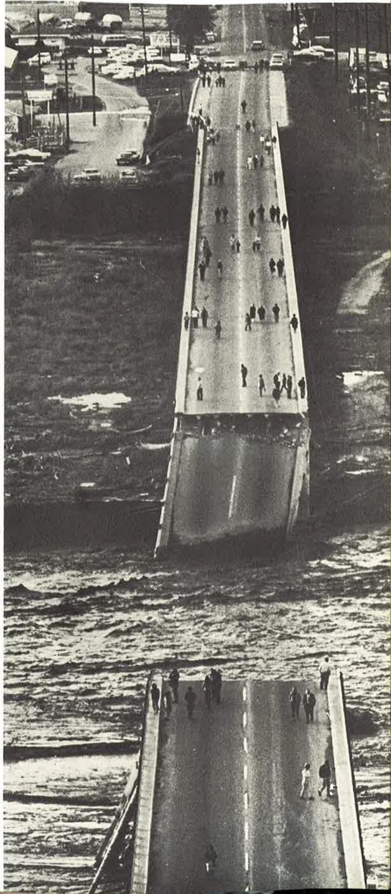
The Highway 118 bridge at Saticoy withstood the January storm, but failed to survive February's onslaught. Motorists, who suddenly discovered they could drive no further, examine the damage.
