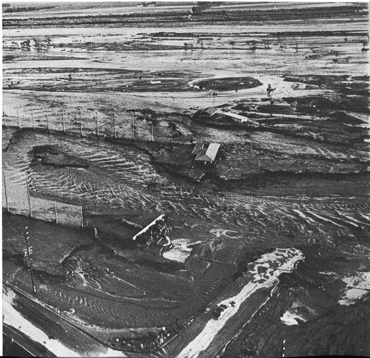
Ventura's new Olivas Park Golf Course, severely damaged by January storms, was wiped out in February. Santa Clara River water, 4½ feet deep, rampages through the pro shop and restaurant. Below, channels up to eight feet deep are cut through the golf course by waters which overflowed the Santa Clara River. In the foreground is the Olivas Park road and the driveway into the parking lot. The course will have to be completely rebuilt.
