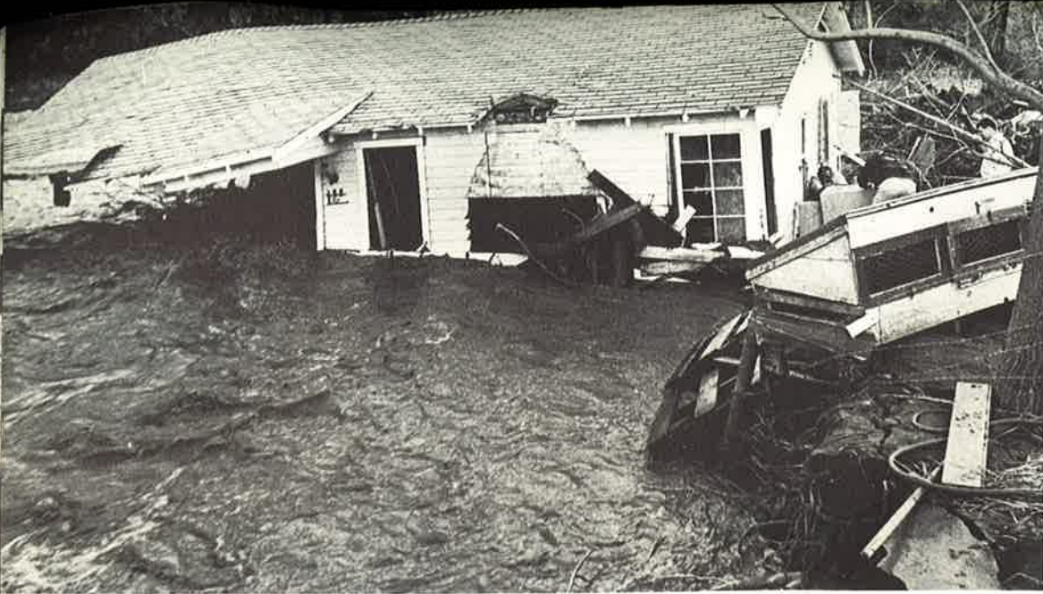
The Creek Road home of Ralph Copus was cut in two and ripped from its foundation by overflowing San Antonio Creek. The dark area of house shows where once the fireplace and chimney were attached.
