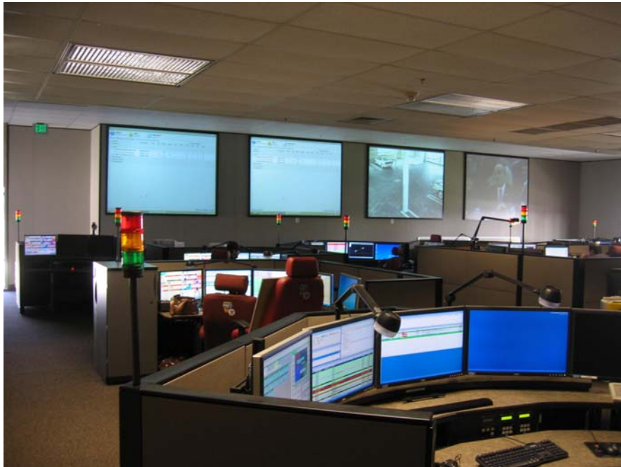
New Fire Communications Center at Camarillo Airport.
