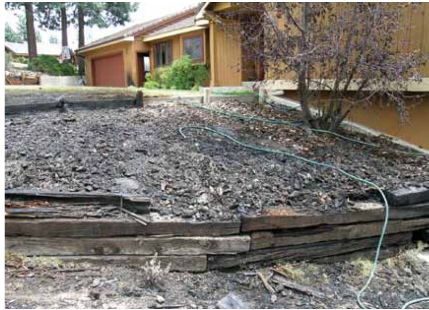
▲ Figure 1. Embers from an oncoming wildfire ignited the pine bark nugget mulch in this flowerbed. The burning mulch then ignited landscape timbers and scorched the adjacent lawn. Fortunately, the house was separated from the mulch by lawn and a concrete sidewalk.
