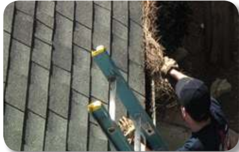
Clear leaves and debris from gutters and check your roof for leaks.
